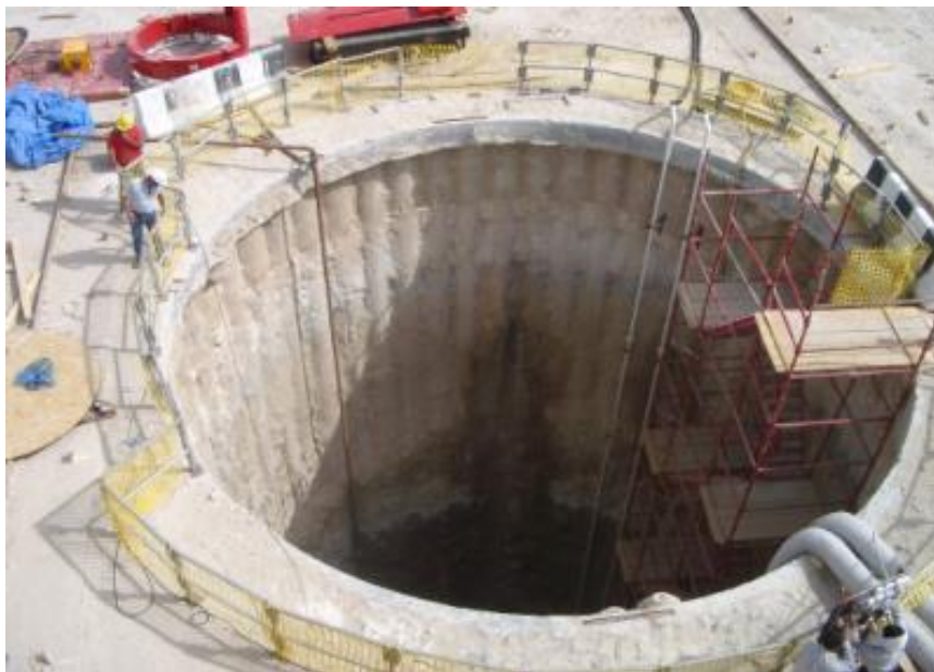
Figure 12 – Shaft being Constructed by Secant Piling Method
